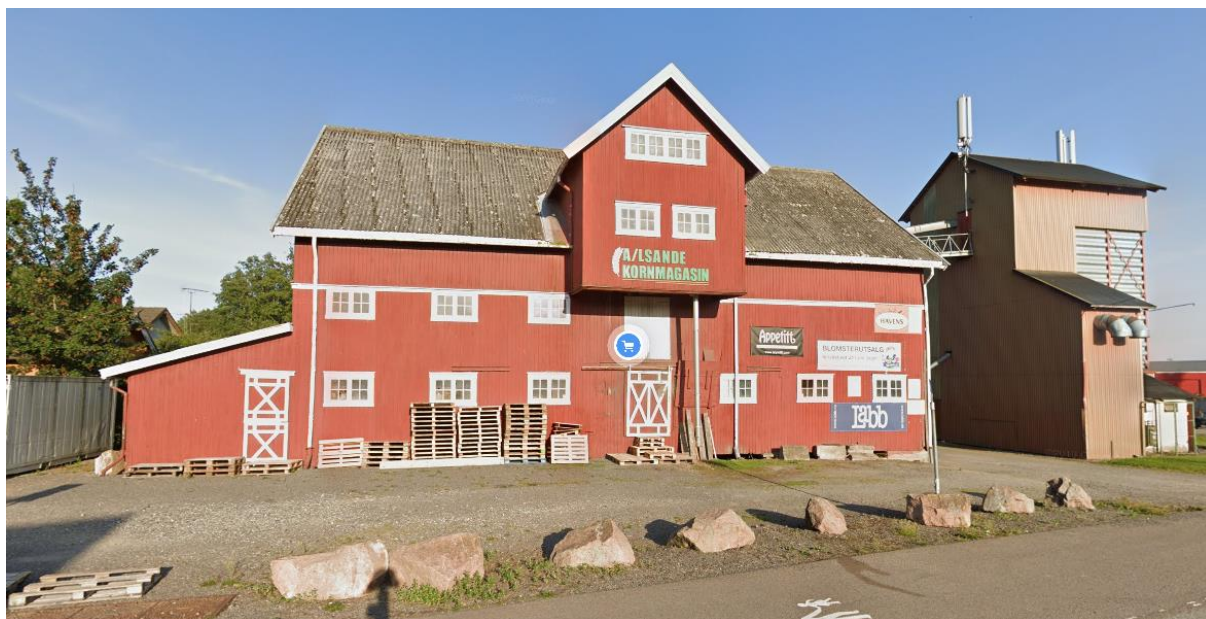
Figur 94: Sande kornmagasin. Foto: Google Street View, august 2019.
